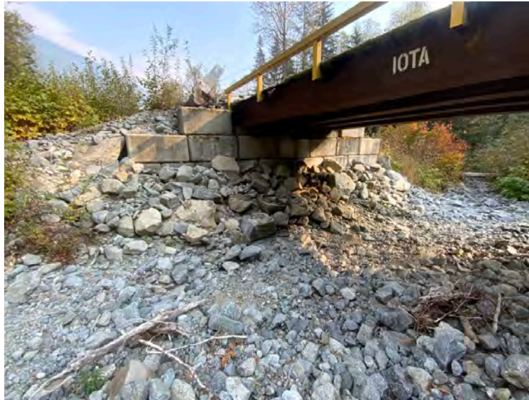
Left Bank Abutment when facing downstream
