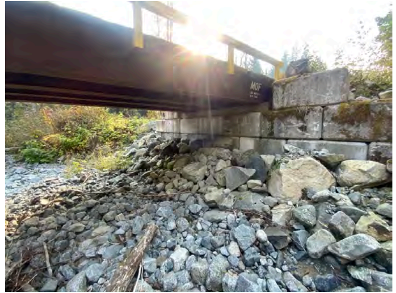
Right Bank Abutment when facing downstream
